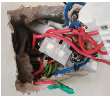
Exposed Conductors
