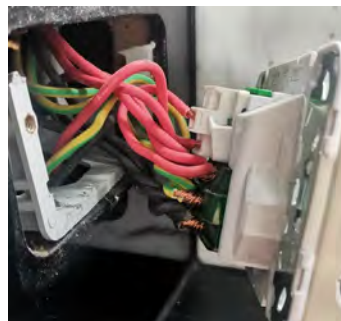
Exposed Conductors
